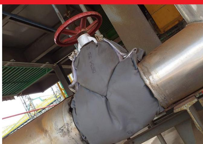
SAIBA COMO REDUZIR AS PERDAS TÉRMICAS DURANTE OS PROCESSOS ISOLANDO VÁLVULAS, CONEXÕES E TUBULAÇÕES!
